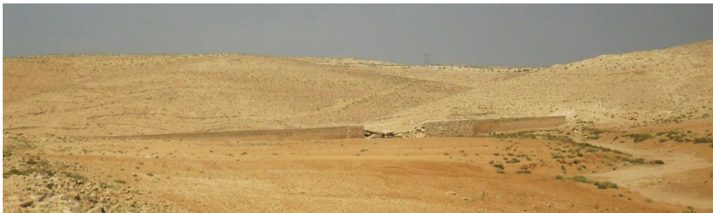
Fig. 4. The downstream dam (Campana, 2011).
