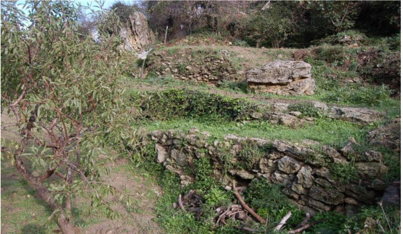
Fig. 13. Connection between terraces at different heights in the Orti Saraceni.
