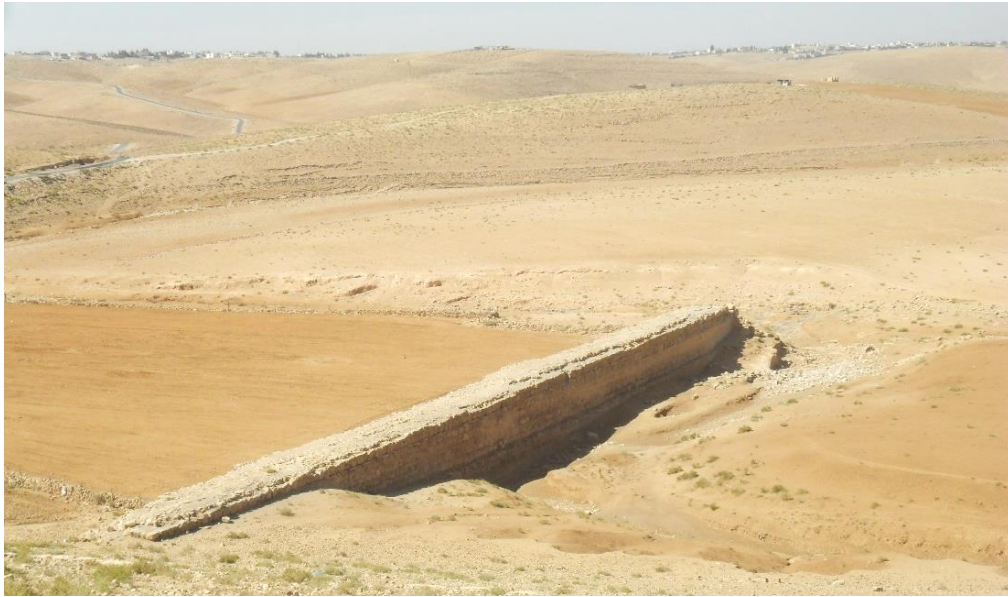
Fig. 1. The upstream dam (Campana, 2011).
